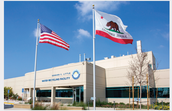
West Basin's Edward C. Little Water Recycling Facility
