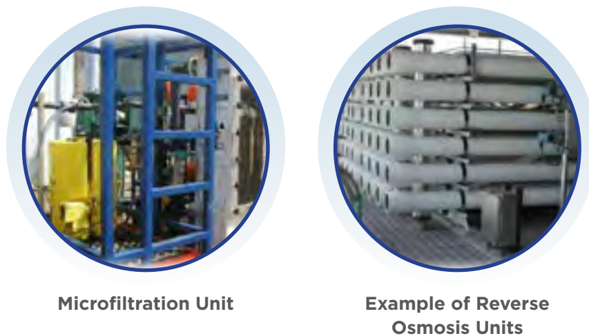
Figure 10-2: Treatment Technologies Used at West Basin’s Pilot Plant
