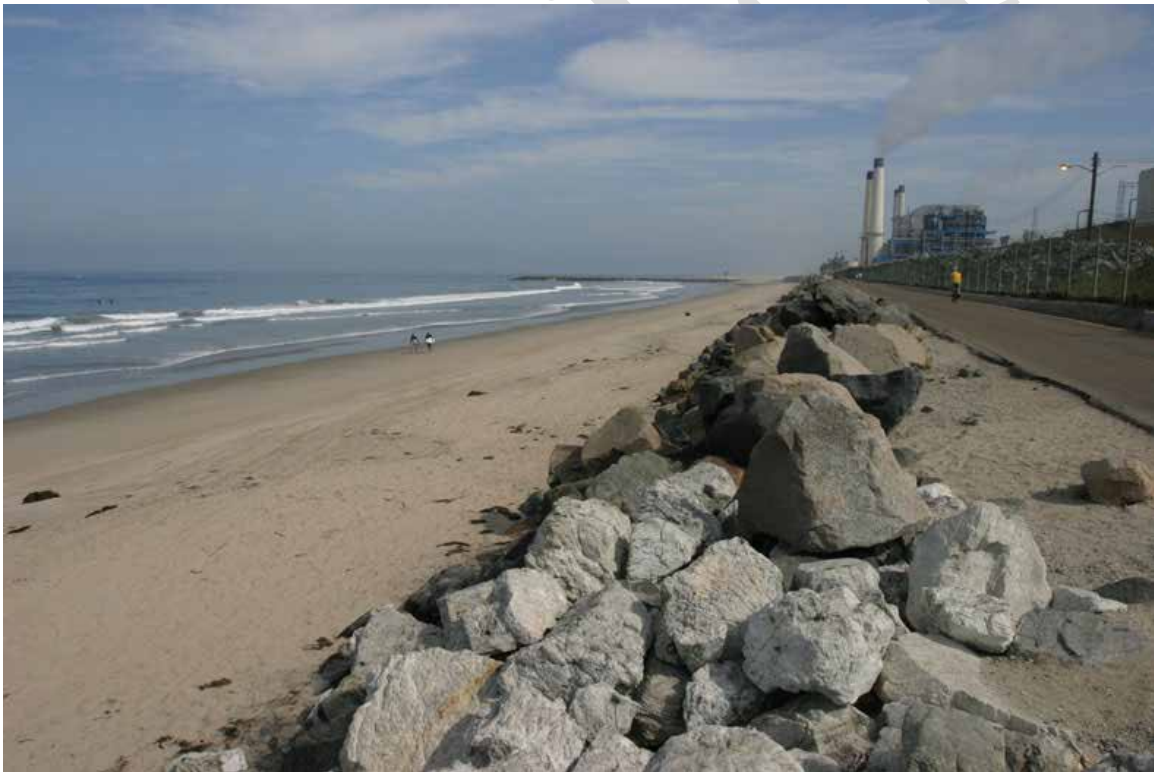
Figure 21. View of El Segundo Beach to the north, NRG El Segundo Generating Station in the background.
