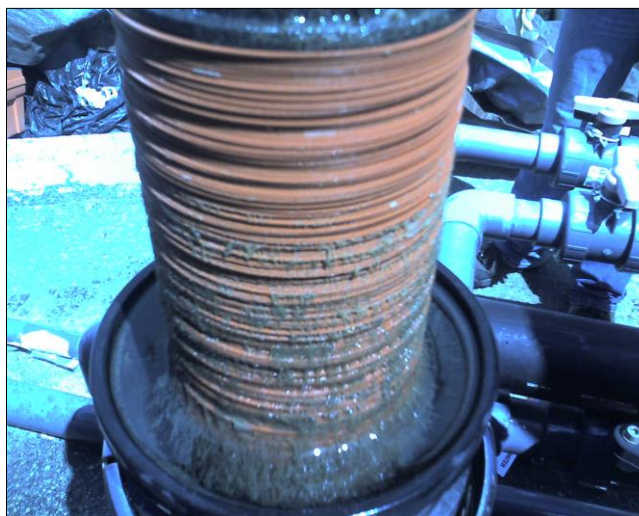
Figure 6-51 Photo of Shells Removed from Arkal Disc Filter Housing
