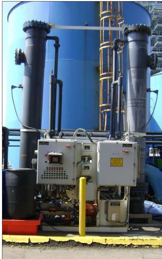
Figure 4-15 High Rate Granular Media Filter
