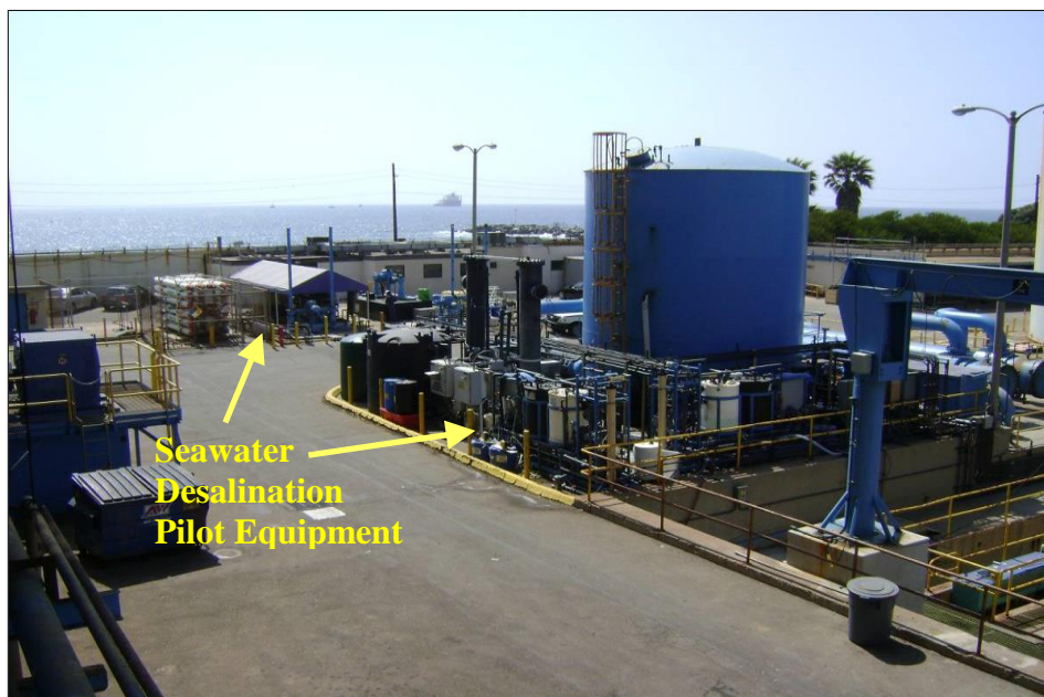
Figure 1-1 Pilot Equipment Onsite at El Segundo Generating Station
