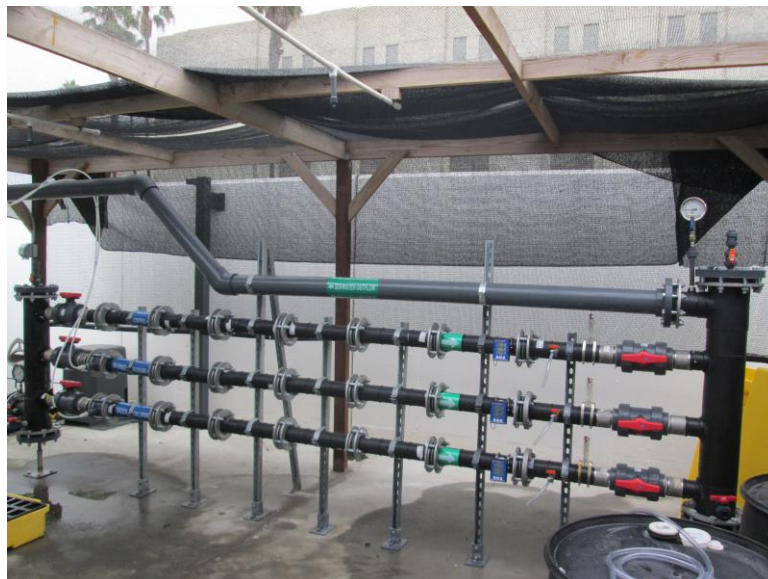
Close-up of the Pipe Test Runs
