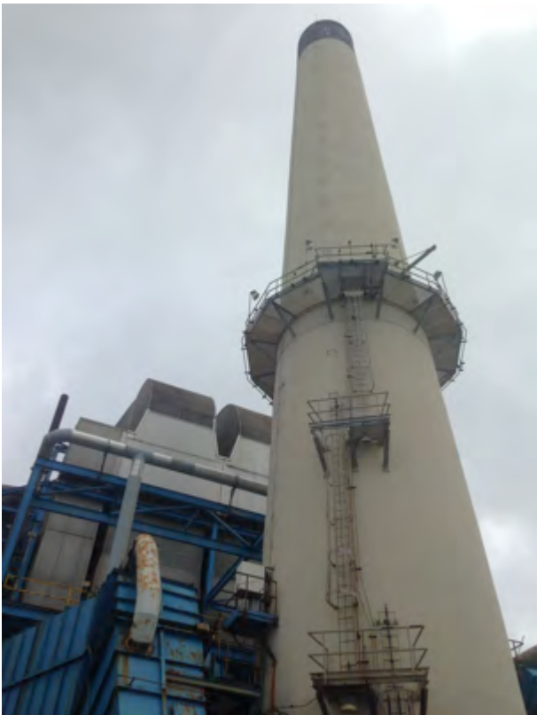
Photo 4: Southern 1964 Smokestack Detail (View Southeast)
