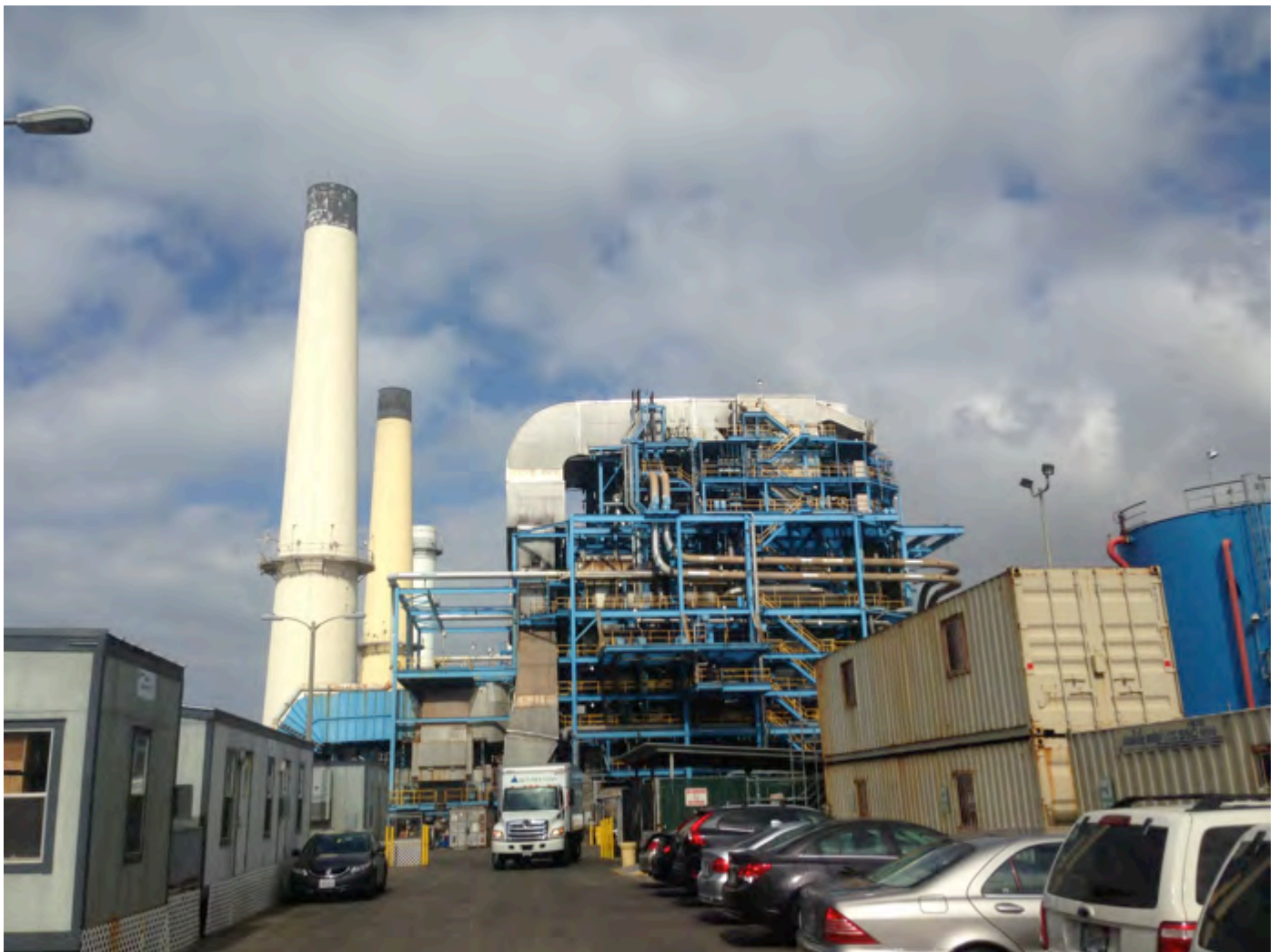
Photo 1: P-19-190098 Overview from South of Smokestacks (View North)
