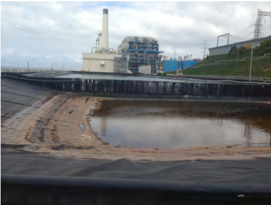
Photo 2: Water Basins Towards Power Plant (View North)
