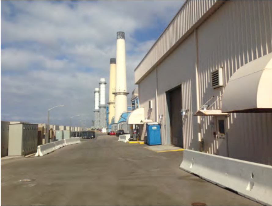
Photo 1: Two 1964 smokestacks in Foreground, two 2012 Smokestacks in Background (View North)
