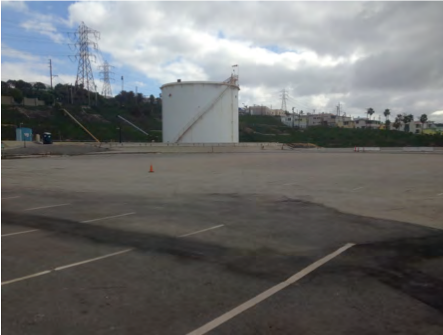
Photo 3: Storage Tank/Parking Lot, and Exposed Sediments (View Southeast)
