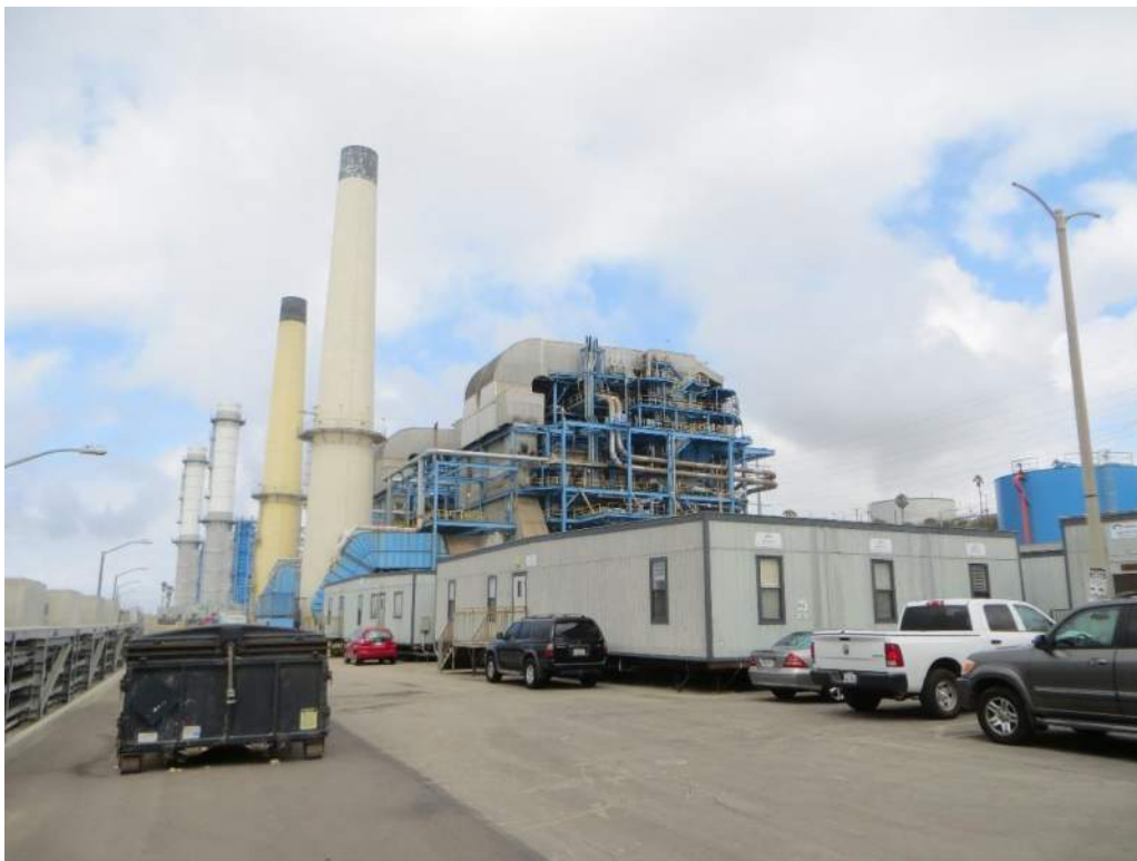
Photograph 6: Most of the project site is a developed steam generation plant.
