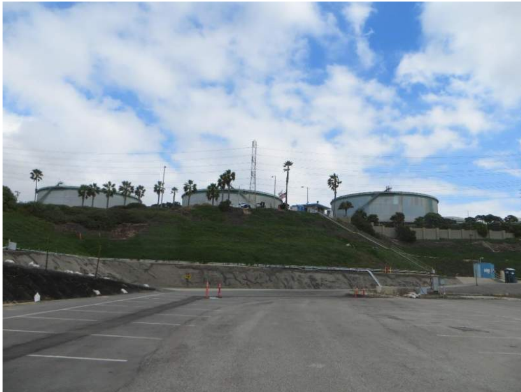
Photograph 4: Facing north from the eastern side of the project site. Most of the vegetation on the site's slopes is ornamental. In this area it is almost entirely ice plant ( Carpobrotus edulis ).
