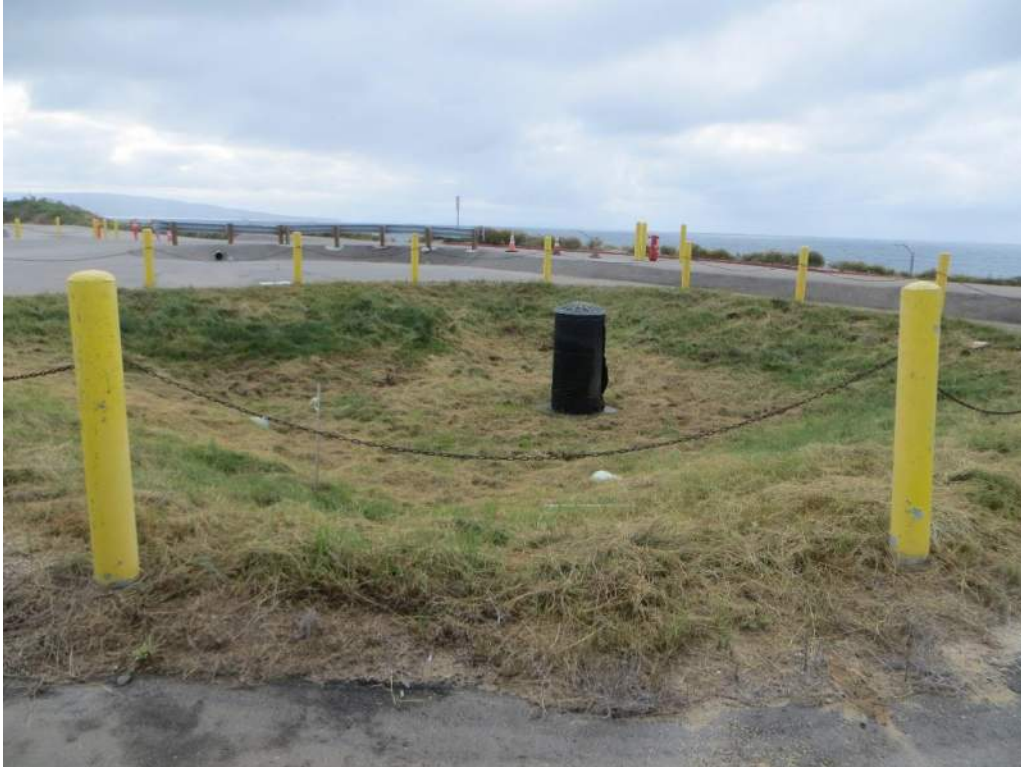
Photograph 5: This water quality basin on the eastern side of the project site does not hold water but is completely covered in grasses.
