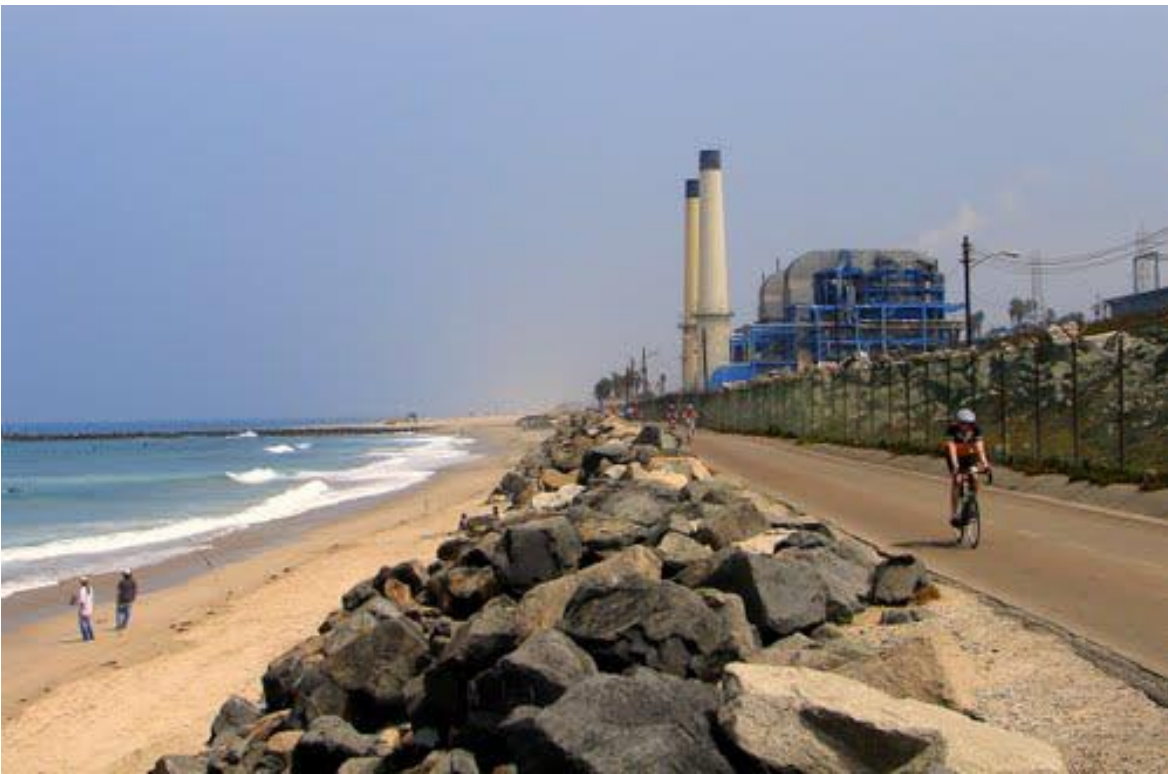
Figure 3: Bike trail perched atop a rip-rap revetment at ESGS site; crest elevation Z = +22 ft to + 23 ft. NAVD
