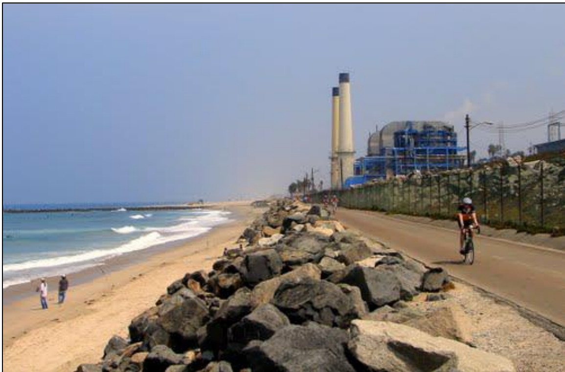
Figure 6.3: Bike trail perched atop a rip-rap revetment at ESGS site; crest elevation Z = +22 ft to +23 ft MLLW
