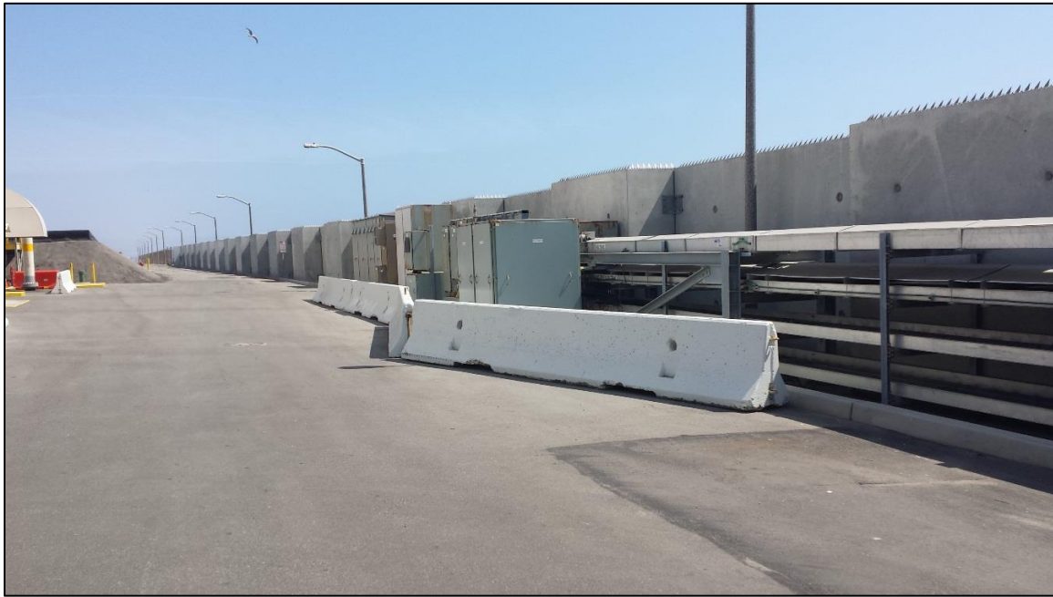
Figure 6.2: Sea wall at the ESGS North Site, crest elevation = + 29 ft MLLW
