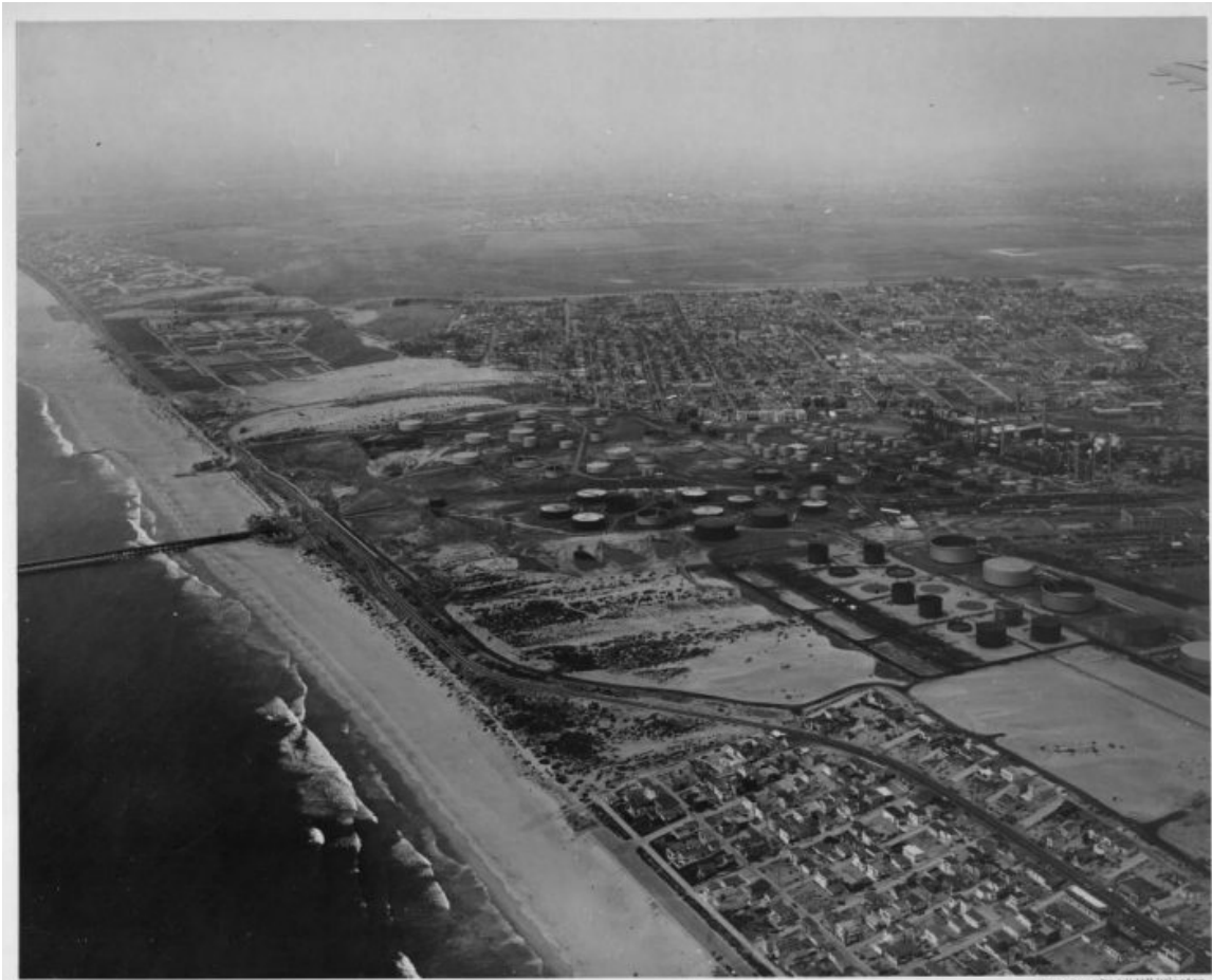
West Basin MWD Ocean Water Desalination Project: Coastal Hazards Analysis / D170766.01 SOURCE: USC Libraries Special Collections, "Dick" Whittington Photography Collection, 1924-1987
