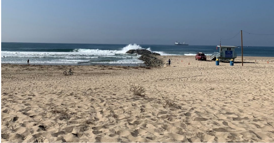
Figure 7 Photograph Showing Difference in Beach Widths North and South of El Segundo Marine Terminal Groin on 10/30/18
