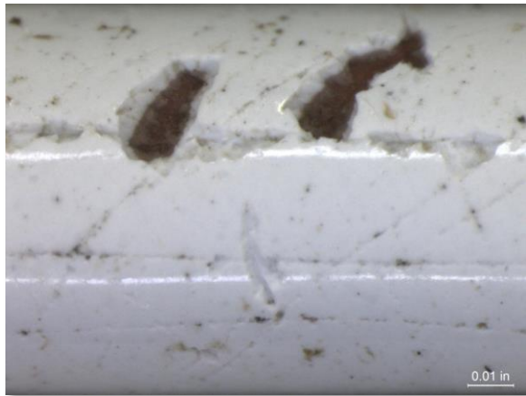
Photo 3-25. 2205 Duplex SS wedge wire screen surface exposed at an area of coating damage.
