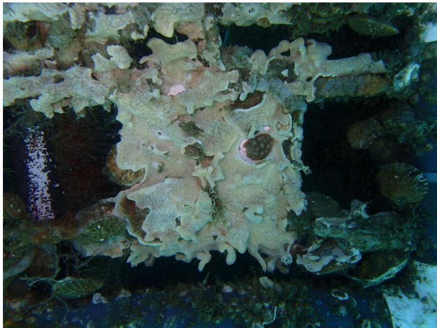
Figure 14. 2205 stainless steel test plate (Test Plate 4), photographed 12/29/14 in situ after removal of its Vexar mesh bag.
