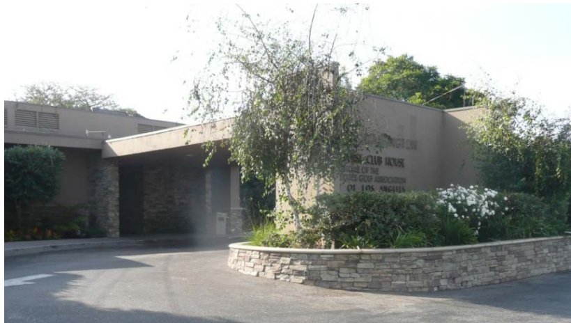
Figure 21. View of Altered Clubhouse, Chester Washington Golf Course SOURCE: Sapphos Environmental, Inc., 2016
