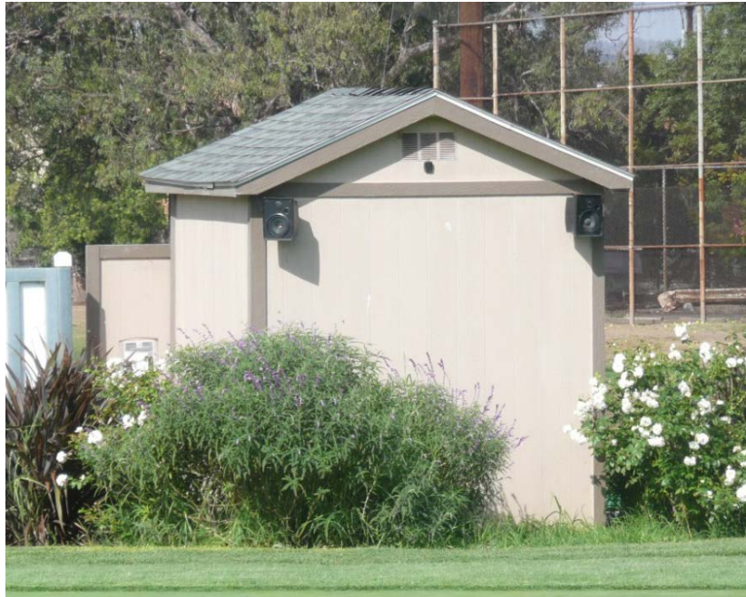
Figure 6. View of Storage Shed, Chester Washington Golf Course SOURCE: Sapphos Environmental, Inc., 2016
